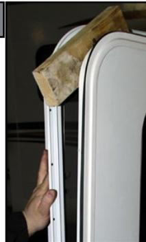
Place a short 2x4, approximately 12-15" long, on a 45-degree angle between the entry door and the door frame at the upper radius. Close the entry door enough to hold the 2x4 in place (Fig. 2).
